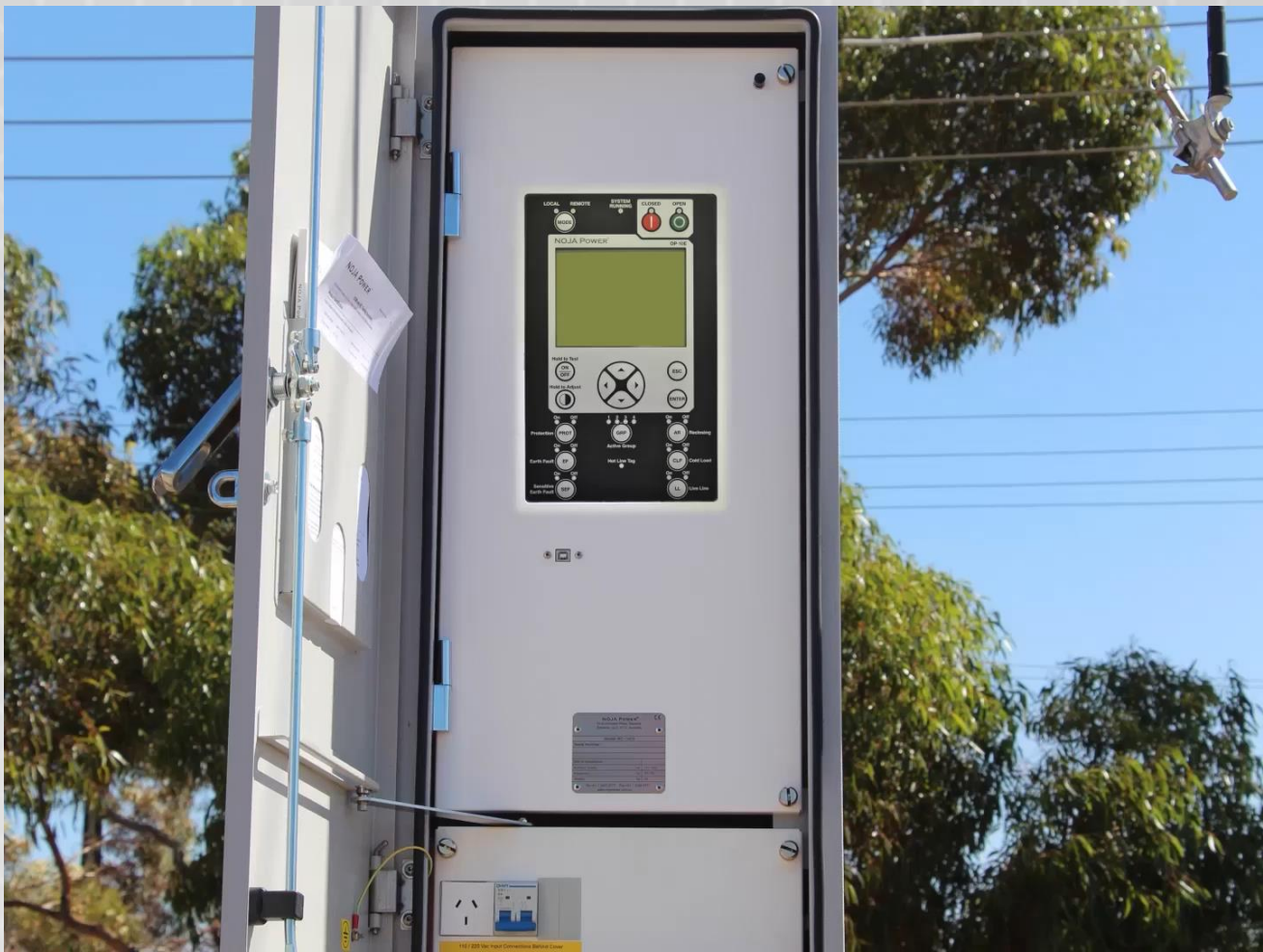
Clip from training movie – “Setting Earth Fault on Noja RC10”
